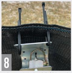
Feed two 75# zip ties through the fabric, into the bracket and back through the fabric.
