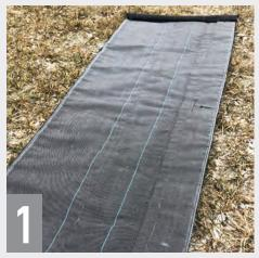
Unroll the silt fence fabric on the ground with the gray panel facing up. The 5" sand tube pocket, with post holes, should be toward the fill slope.
