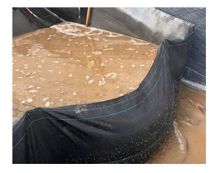
Self-supporting onion tank design provides at least 380% more tipping stability compared to super silt fence.
