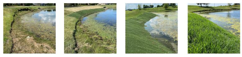
Eroded, undercut pond and lake banks are difficult and dangerous to maintain and use. The InstaTurf® simulated turf structure and specially engineered filtration fabric work together to stabilize shorelines by preventing soil/seed migration and extraction under wave action and fluctuating water levels.
