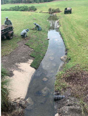
EXHIBIT 1: Typical DredgeSOX Installation (Source: SOX Erosion Solutions)
