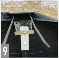
Tighten zip ties. The fabric will not be tight horizontally or vertically to allow the selfsupporting curve to function.
