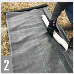
Insert sand tubes into tube pockets between the post holes in the fabric.
