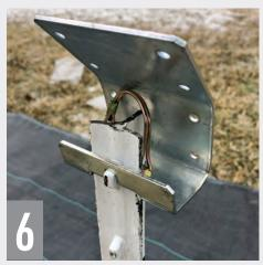
Place angled top bracket on top of T-posts and pin into place. Ensure that the open side faces the fill slope.
