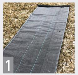
Unroll the silt fence fabric on the ground with the gray panel facing up. The 5" sand tube pocket, with post holes, should be toward the fill slope.
