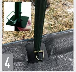
Drop bottom plate over end of post and place retainer clip on top. Finish driving T-post until bottom plate is tight and flush with ground, sealing tube pockets in place.
