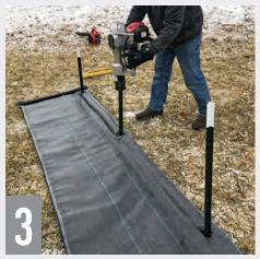
Start T-posts in holes between sand tubes (studded side facing fill slope), with the white end facing up. Set with a driver, pounder or sledgehammer.
