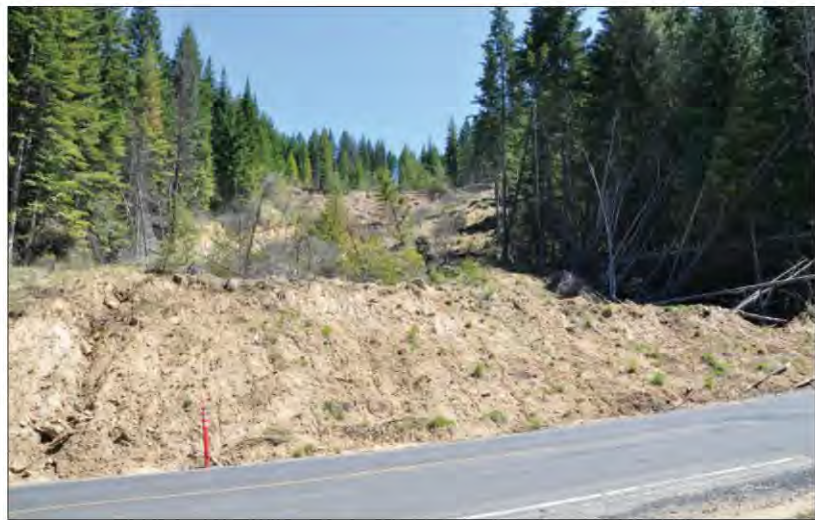
A massive landslide occurred as a result of intense runoff, causing significant damage to the road infrastructure and surrounding slopes.
