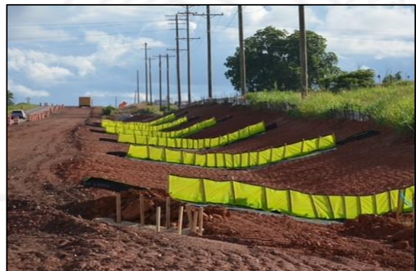
Natural floatables contribute to filtration on green mesh of velocity restrictor sheet
