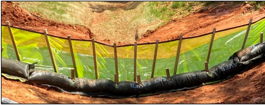
High Velocity Geotextile Ditch Check System showing front water seal with compression tubes and stakes
