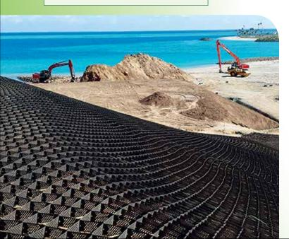
GEOWEB® slope protection systems may be designed with a variety of infill materials to meet project requirements for aesthetics, stability, environmental impact, material availability, and erosion-control. The system also provides protection to impervious liners.
