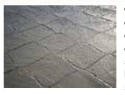
GEOWEB<sup>®</sup> slopes with concrete infill provide economical, hardarmored protection of slopes exposed to severe hydraulic or mechanical stresses. The quality,
