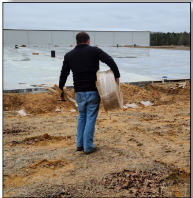
WattleFence installed (top), 200 linear ft of WattleFence can easily be carried on a project site (bottom).
