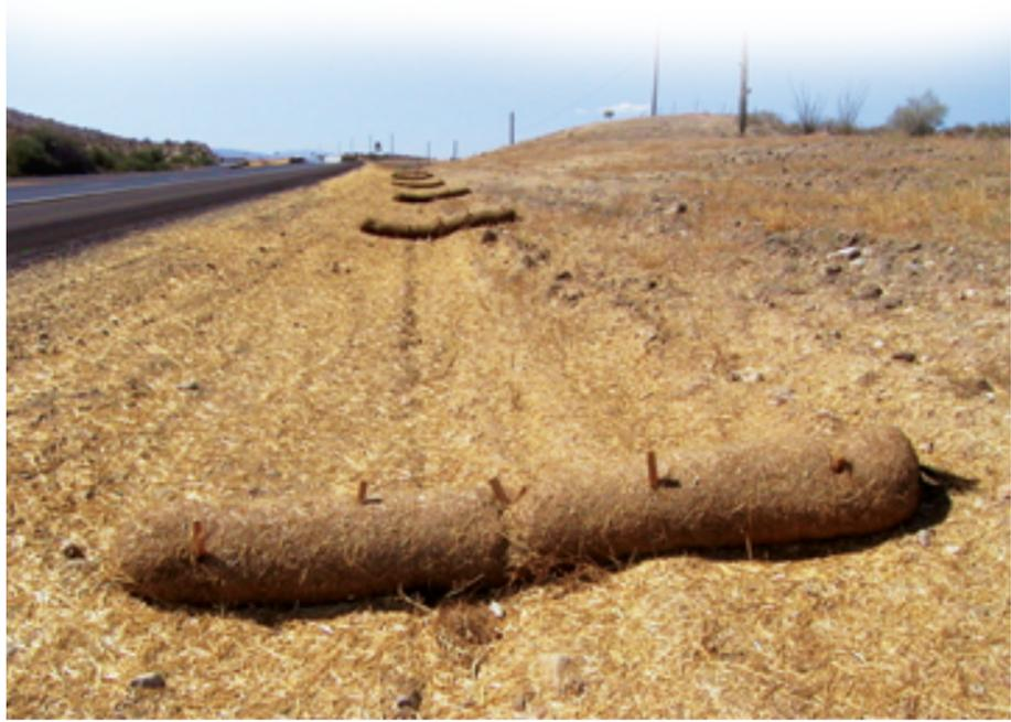
Excel Straw Logs consist of a 100% straw matrix confined by a tubular synthetic net. Excel Straw Logs function well as low-flow inlet filters and roadside filters, as they allow minimal flow and sediment to pass through. The logs are flexible, conform to the soil surface, and are secured by staking.
