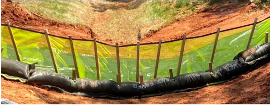
High Velocity Geotextile Ditch Check System showing front water seal with compression tubes and stakes
