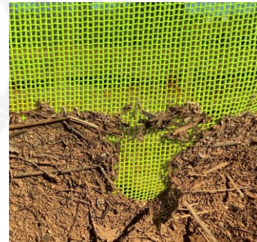
Natural floatables contribute to filtration on green mesh of velocity restrictor sheet
