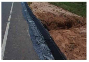
The 5" Triangular Silt Dike™ barrier was designed for smaller flatter runoff areas. It has a protective apron on the front or upstream side of the barrier. With no protective apron on the backside or downstream side, this should be installed along curbs or on hard surfaces where overtopping the barrier will not cause erosion on the backside.
