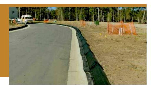
The 5" Barrier is the Better solution to silt fence, sand bags, and straw wattles!
