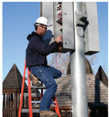
Having major electrical components accessible at ground level avoids hiring a $100/hour crane to replace a $10 fuse.
