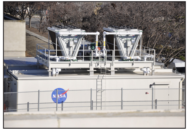
The Electra supercomputer is a petascale proof-of-concept system for the agency's modular computing technology, which saves significant amounts of water and power annually. Marco Librero, NASA Ames
